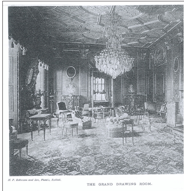
Fig. 5: Grand drawing room, Lynford Hall, 1895, photograph taken from the Lynford Hall Estate sales brochure, private collection.
